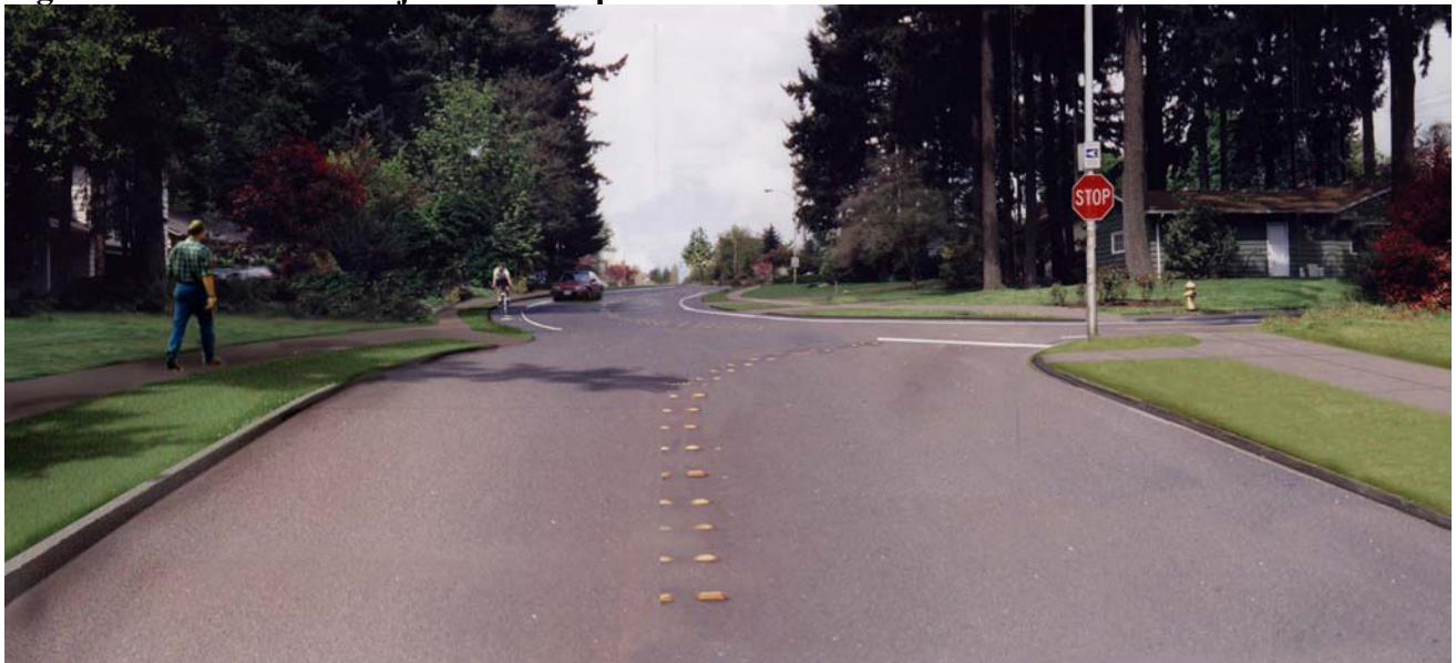
Figure 6-8: Road Diet Project After Improvement
