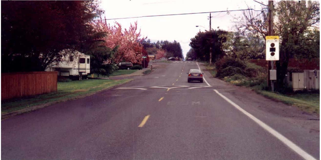
Figure 6-1: School Crossing Before Improvement
