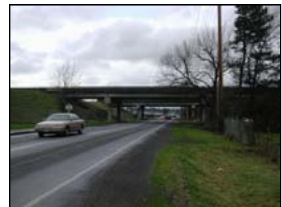
Burton Rd. underpass at I-205
