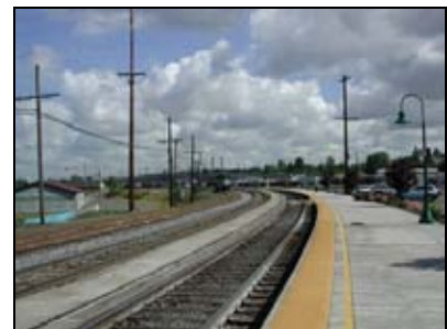
Rail alignment at Amtrak station
