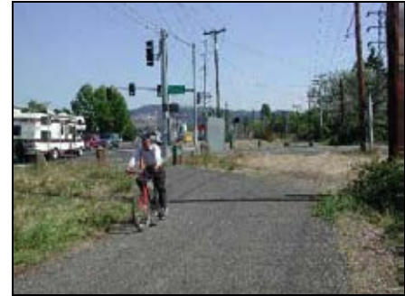
Type 2 treatment on Springwater Corridor, Portland
