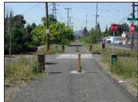
Type 1 treatment on Springwater Corridor, Portland
