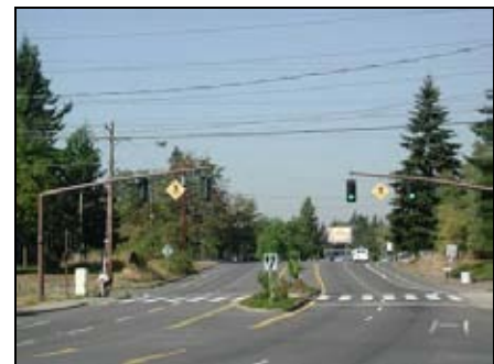
Type 3 treatment on Springwater Corridor, Portland
