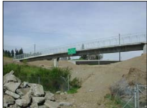
Overcrossing of I-5
