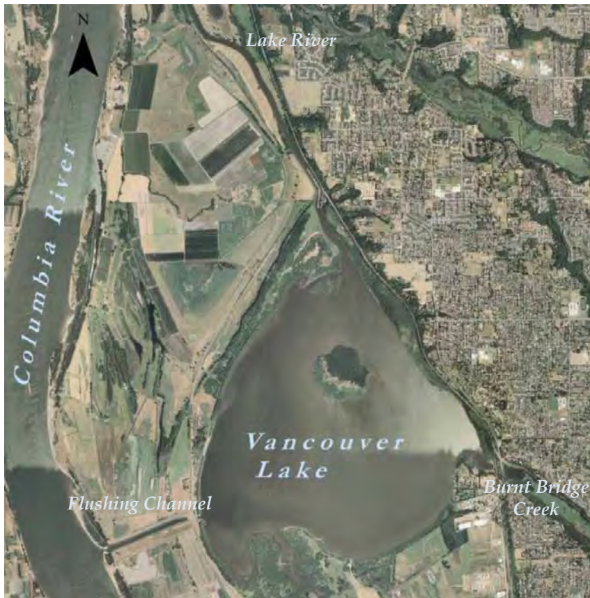
Figure 2-1: Flushing Channel, Lake River, and Vancouver Lake
